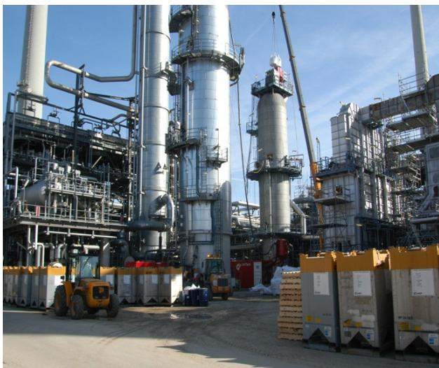
for removing sulphur from gasoline and diesel to produce cleaner fuels and as in the case of the CHD are often on the 'critical path' of a larger refinery turnaround. Historically the unit has experienced unloading problems during its catalyst changeout including high concentrations of flammable vapours or LEL and agglomerated catalyst.
